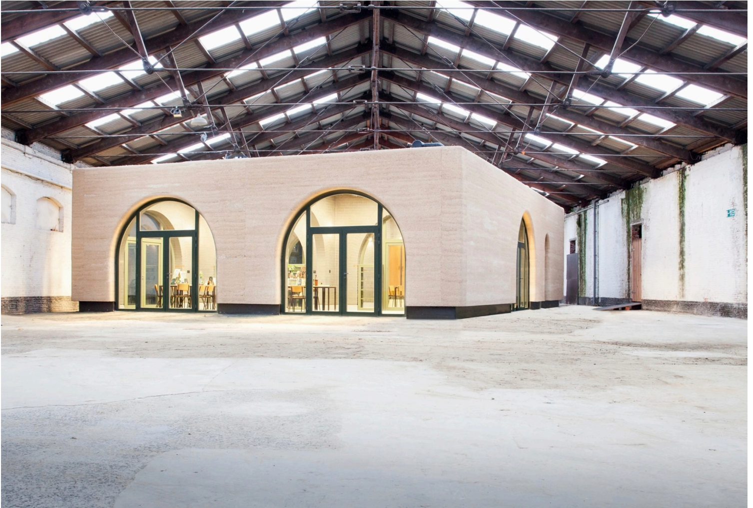
Regional House Edegem, BC architects
