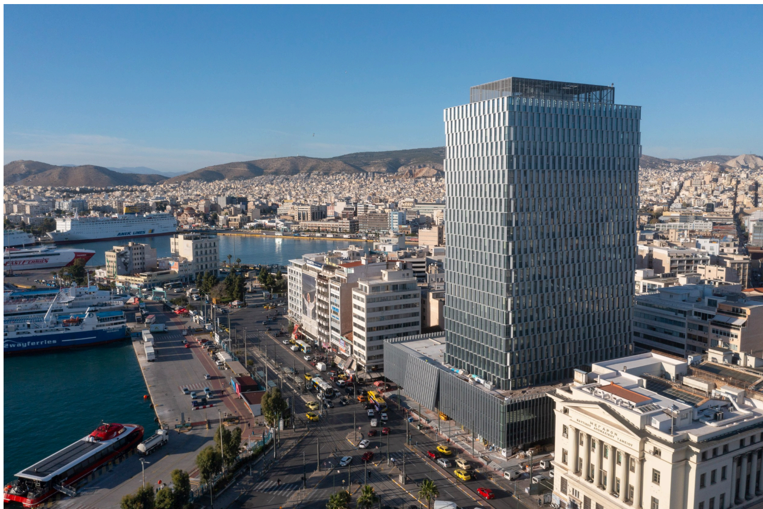
PIRAEUS TOWER, DESIGN BY PILA | Photos ©NikosDaniilidis
