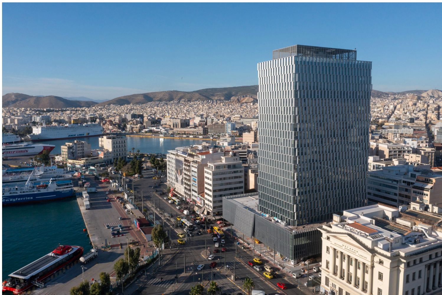
PIRAEUS TOWER, DESIGN BY PILA | Photos ©NikosDaniilidis
