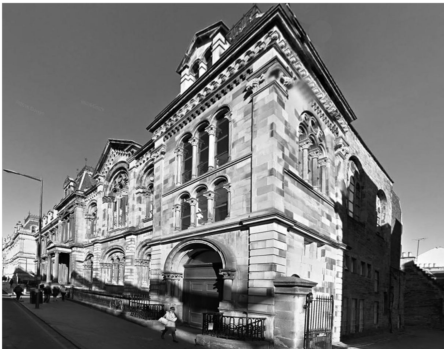
Εικ.15 Minto House, Chambers Street
