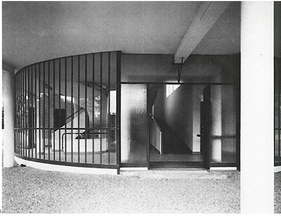
29. Villa Savoye entrance: beam from column in foreground meets beam between columns inside that flank door, thus articulating entry. Straight ahead is the ramp. 30. entrance hall with ramp on right and service stairs on left. 31. first-floor terrace, looking away from living room. 32. at head of ramp on first floor looking past service stairs towards Madame's bedroom.
