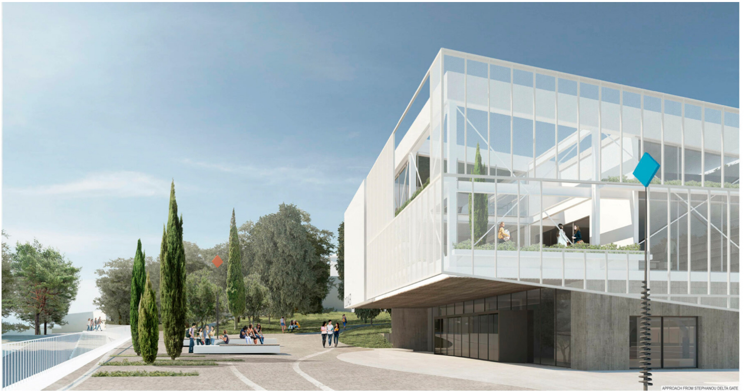
APPROACH FROM STEPHANOU DELTA GATE
