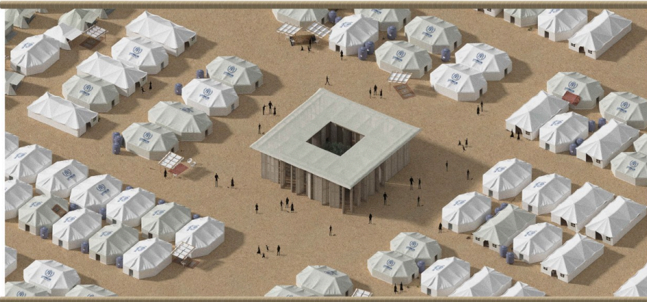
1. Roof: Protective waterproof canvas is only non paper material
